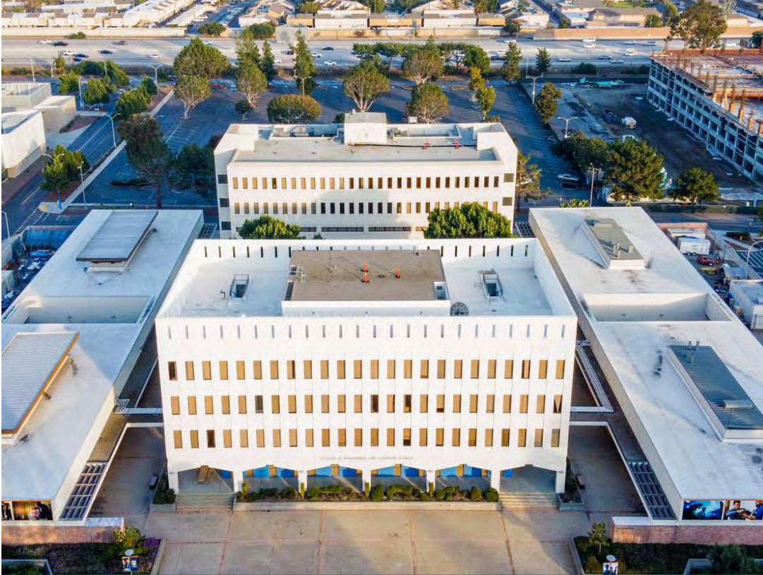
Existing Engineering and CS Buildings
